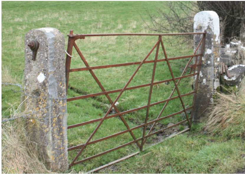
Typical Pollok field-gate and piers
